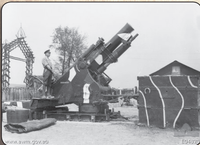
The 185th was a siege battery equipped with heavy howitzers sending large calibre high explosive shells in high trajectory plunging fire. A British soldier standing with a 9.2 inch howitzer Mk 1 which supported the Australians on the Somme.
